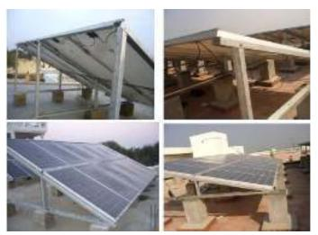
Figure 4.7: GI mounting structure
